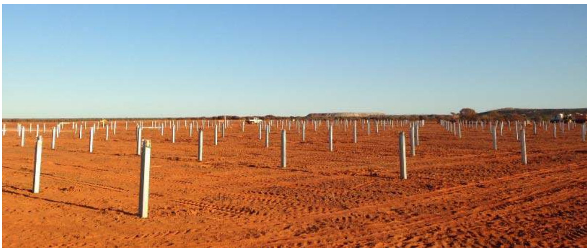
Figure 3-6 Example of poles driven into the ground on a Neoen solar project in Western Australia
