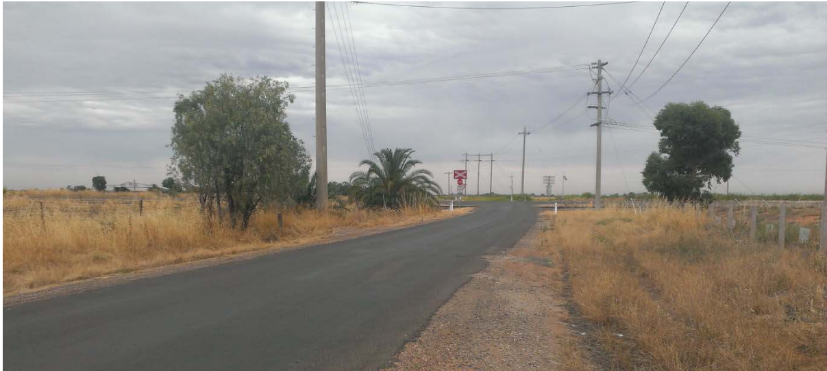
Figure 3-5 View of Hamilton Road toward Irrigation Way with the railway line level crossing visible
