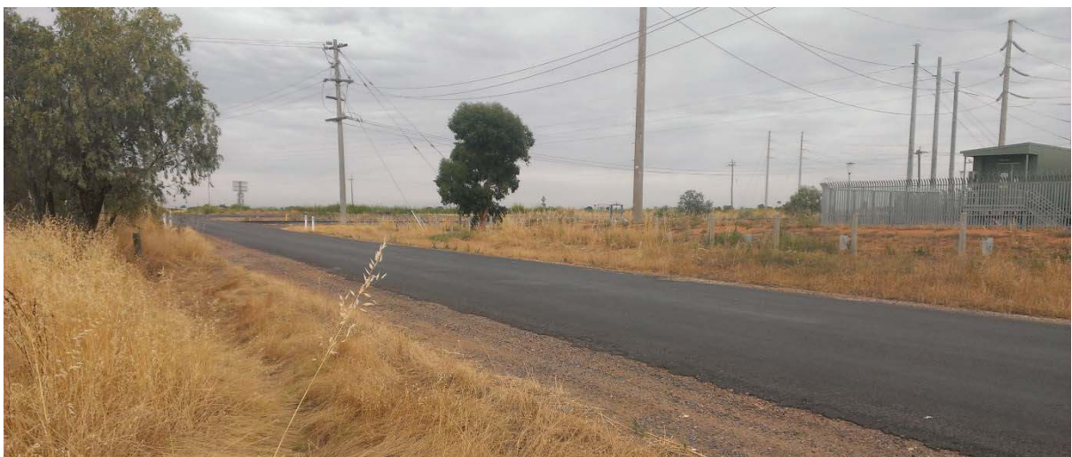
Figure 3-4 View of Hamilton Road and Transgrid substation
