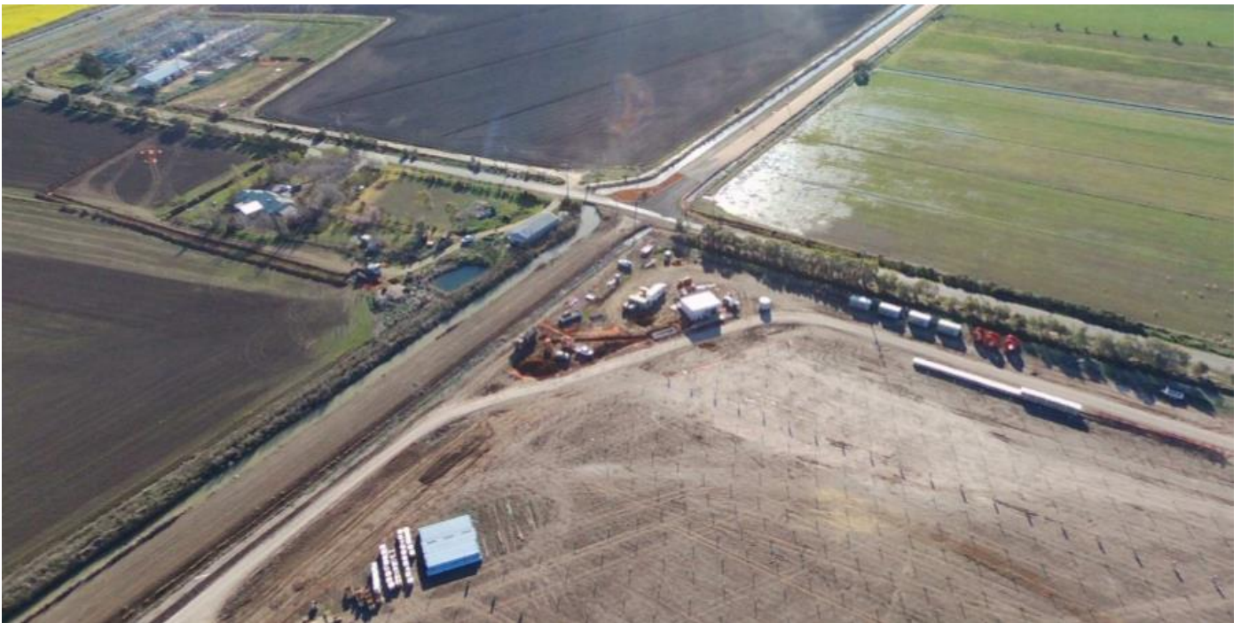
Connection to the grid
